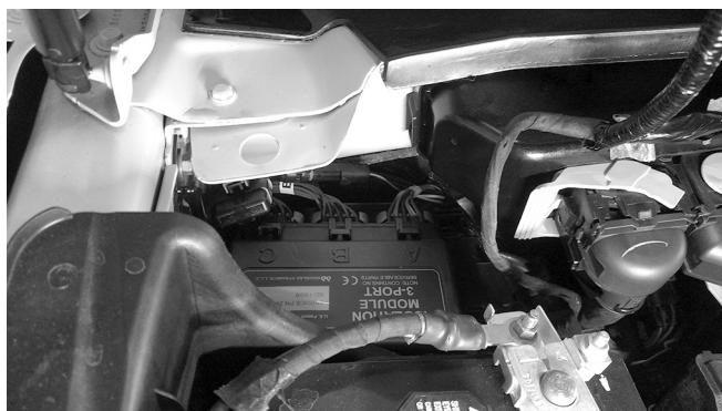
Isolation module, after installation.
